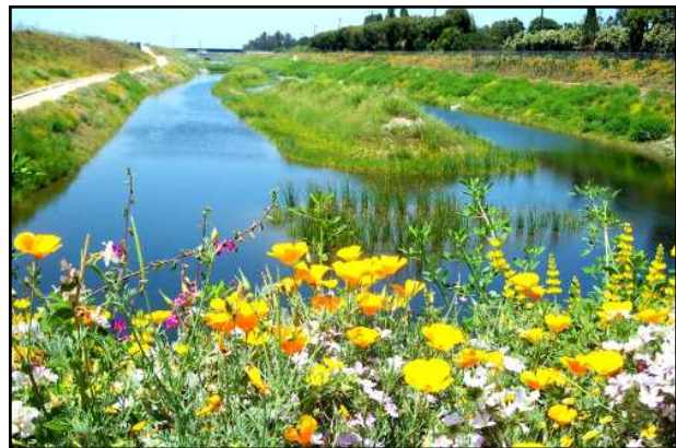
Post-Construction Photo: Wetlands
