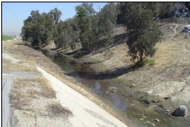
Pre-Construction Photo: Spreading Ground Basin
